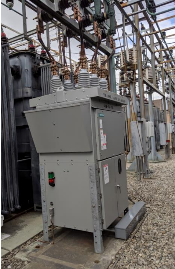
New 4kV VCB
