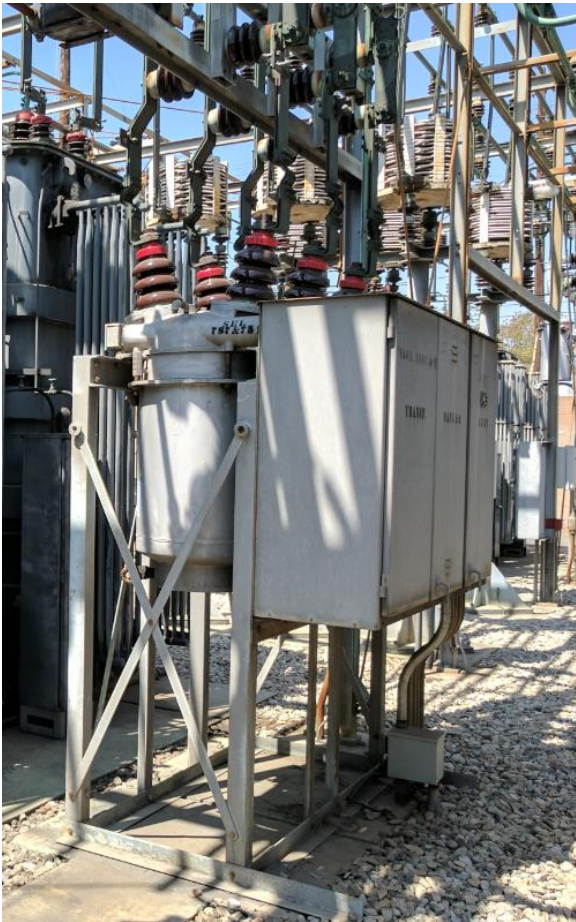
Original 4 kV OCB
