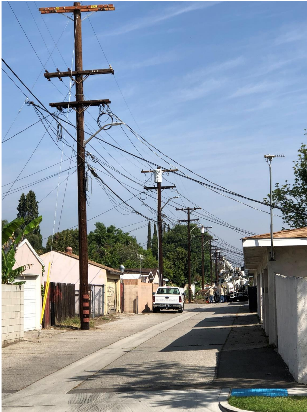
N-15 Alley Work
