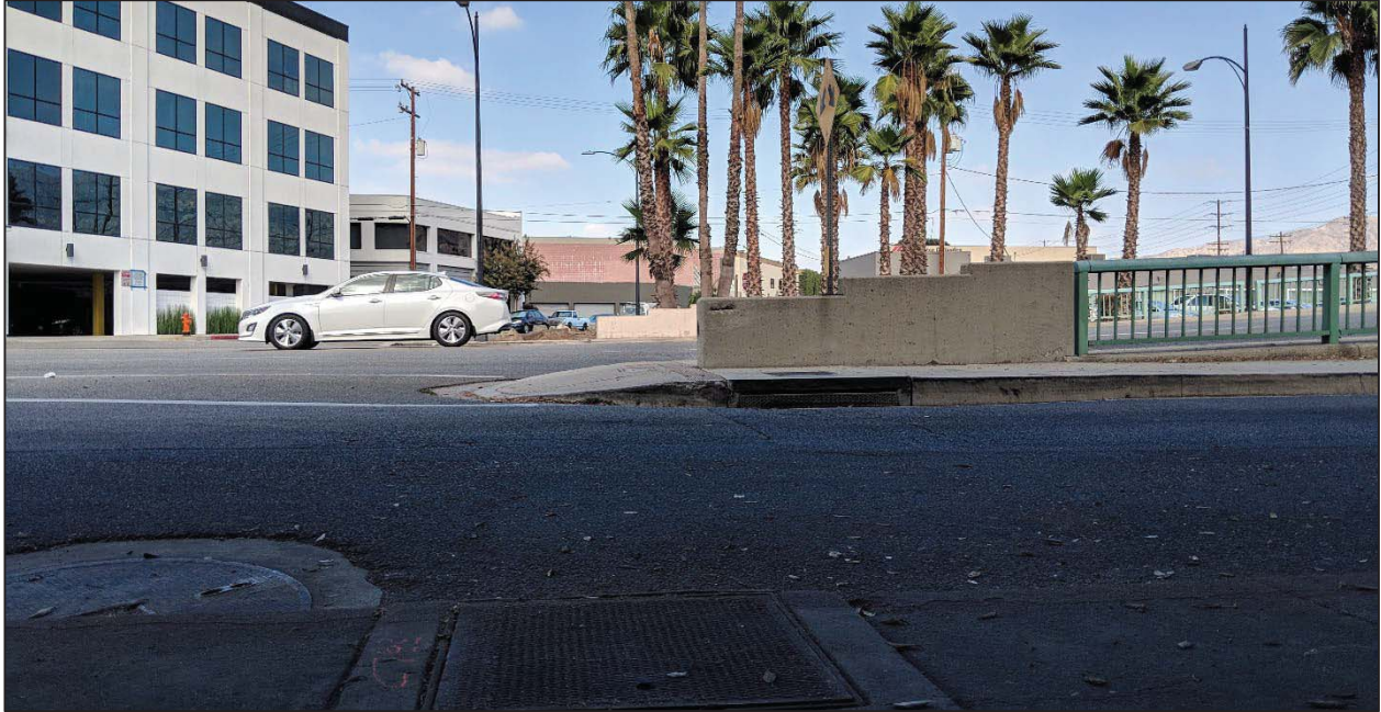
Photograph 1: Representative photograph showing location of current stormwater system currently connecting adjacent property to Project Site
