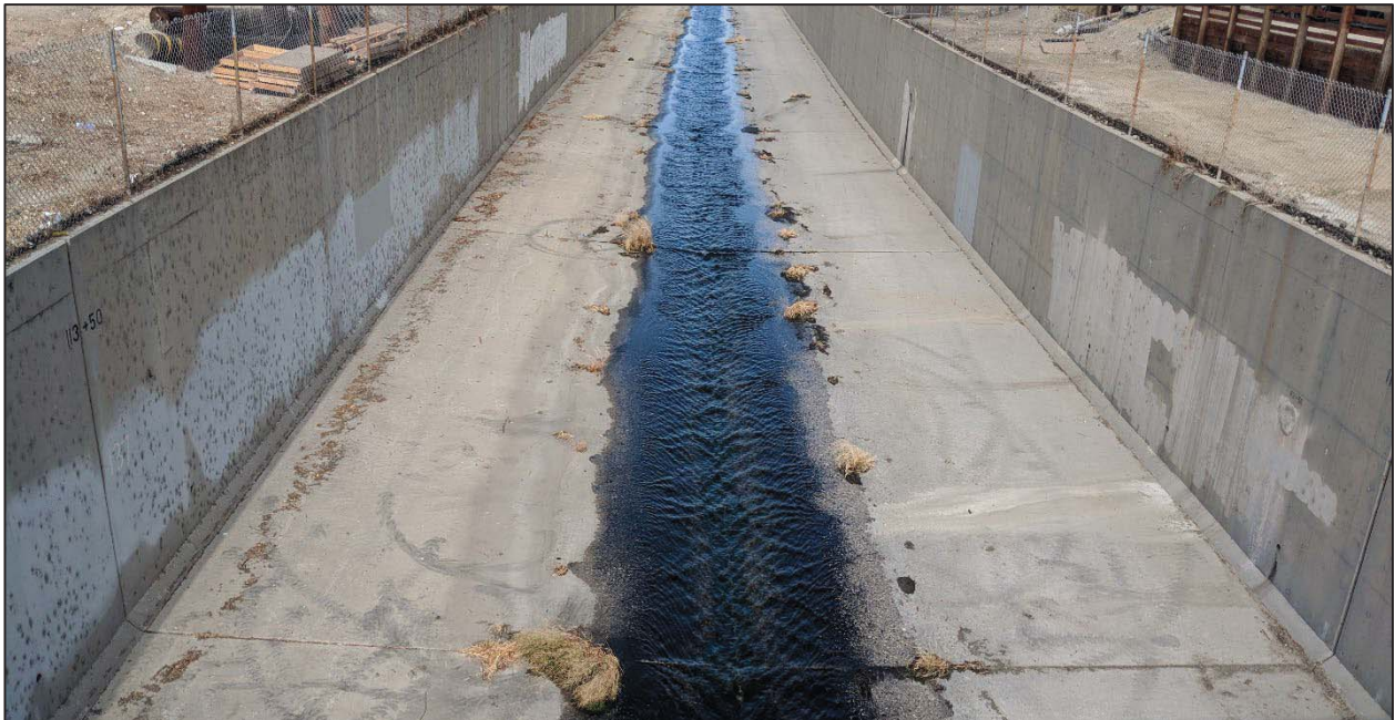
Photograph 2: Representative photograph showing the Burbank Western Channel
