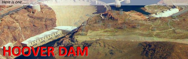
Few power generation facilities are as iconic or inspire as much awe as the Hoover Dam. First envisioned in the early 1900s and constructed between 1930 and 1935 during the Great Depression, the Hoover Dam produces power using 17 hydroelectric turbines rated at 2,080 megawatts (MW) in aggregate. Hoover Dam straddles the Arizona-Nevada border, with one set of turbines on the Arizona side and the other set on the Nevada side.
