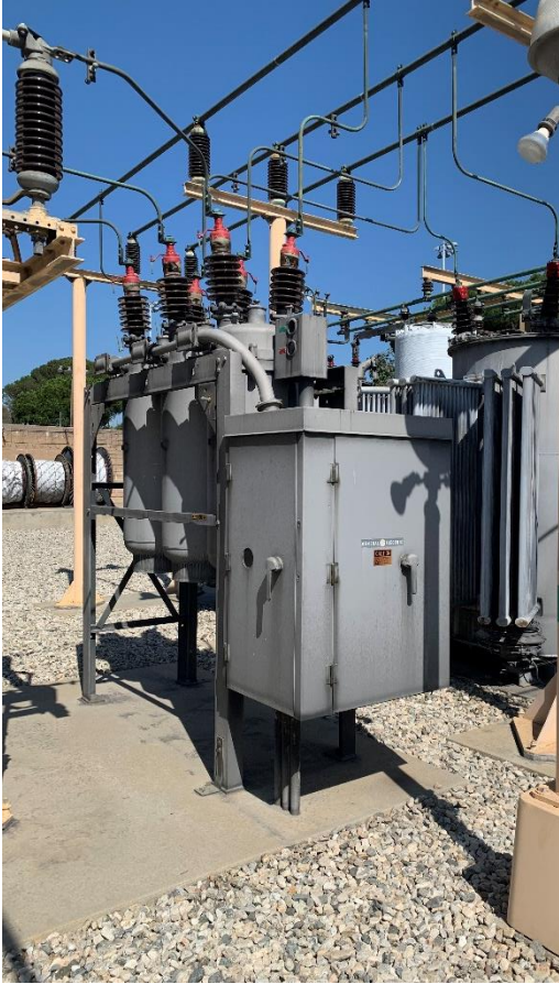
Old 34.5kV OCB
