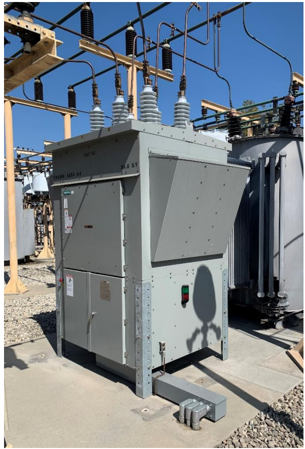
New 34.5kV VCB
