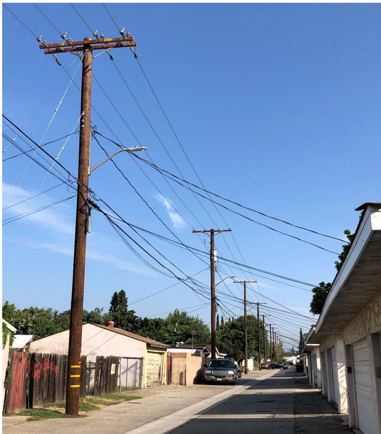
Completed N-15 12kV Alley Work E/O Catalina St.
