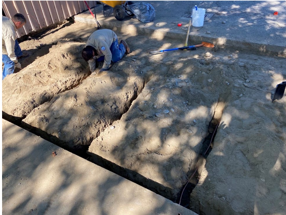
Ground Grid Work at Victory Substation
