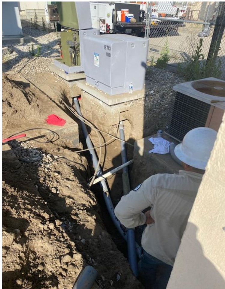
Conduit Work for the AC Power at Olive Sw. Substation
