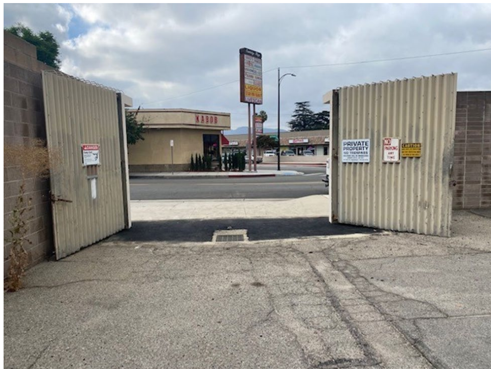
Asphalt Addition Work at McCambridge Substation
