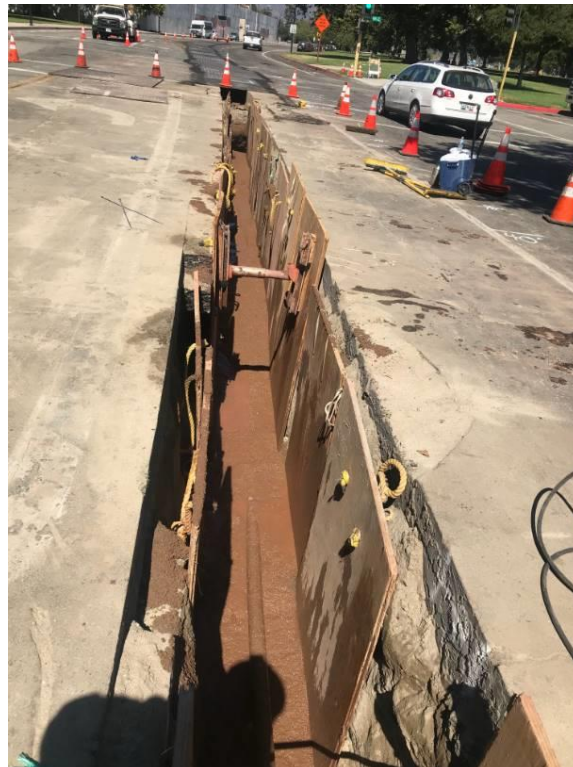
Underground trench for electric conduit installation
