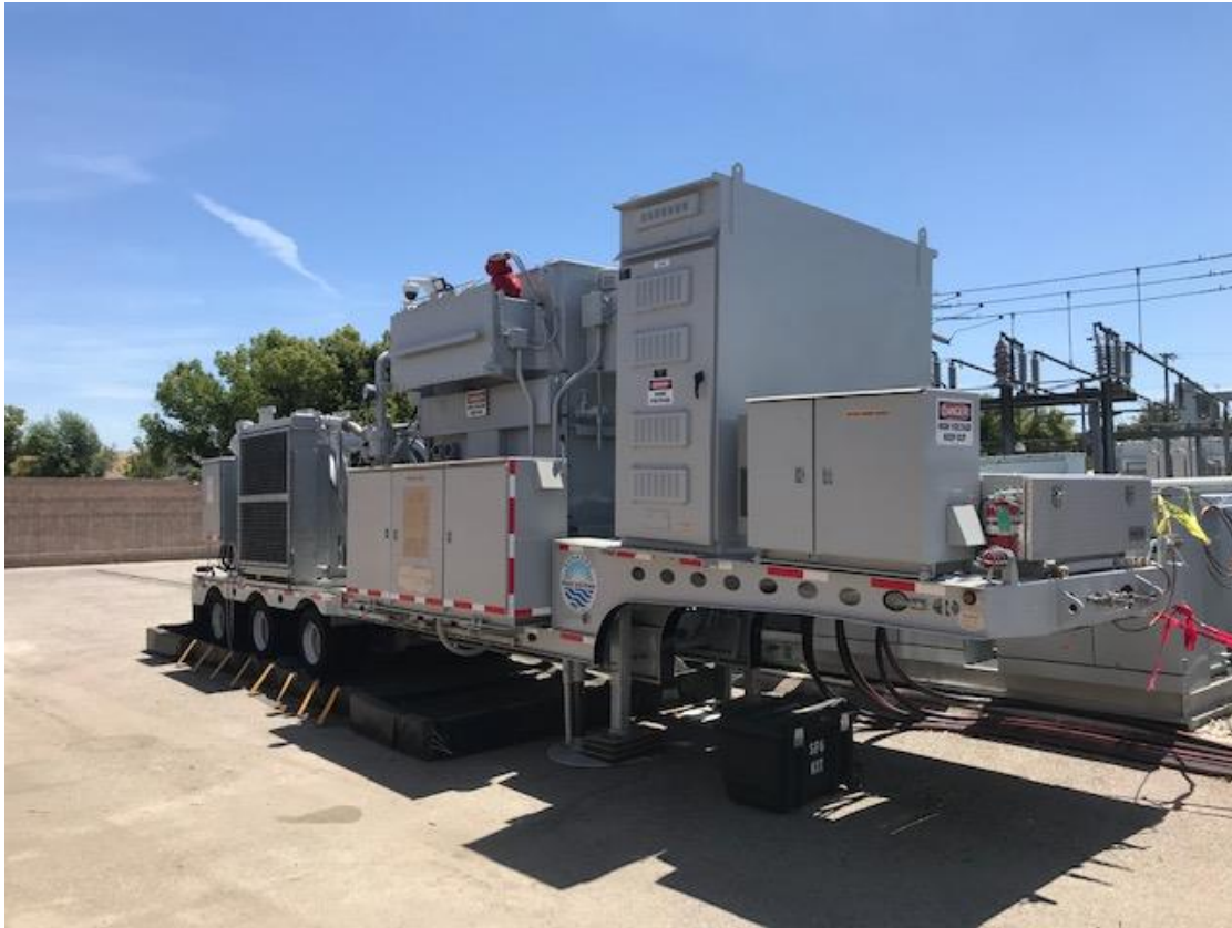
Mobile Substation at Golden State Substation
