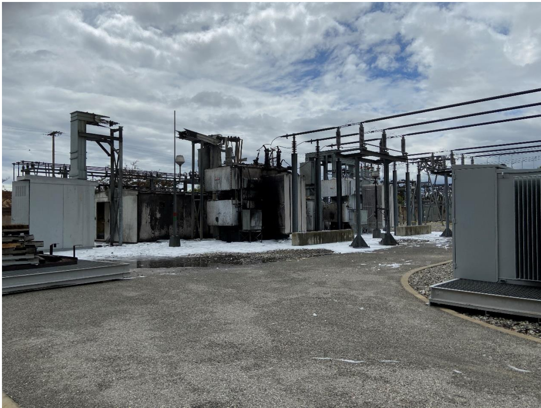
Golden State Substation After Transformer Fire on 4/10/2020
