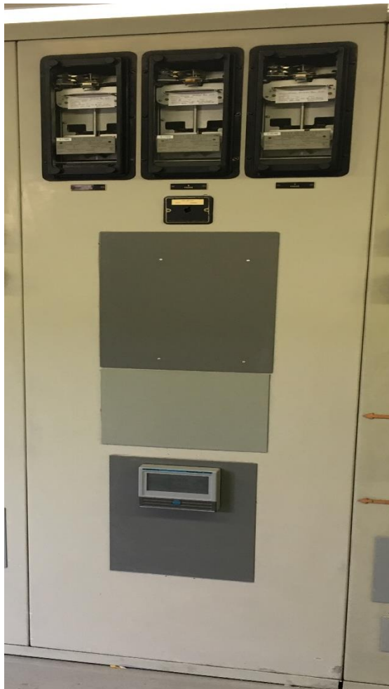
Bus Diff. Relays before Replacement
