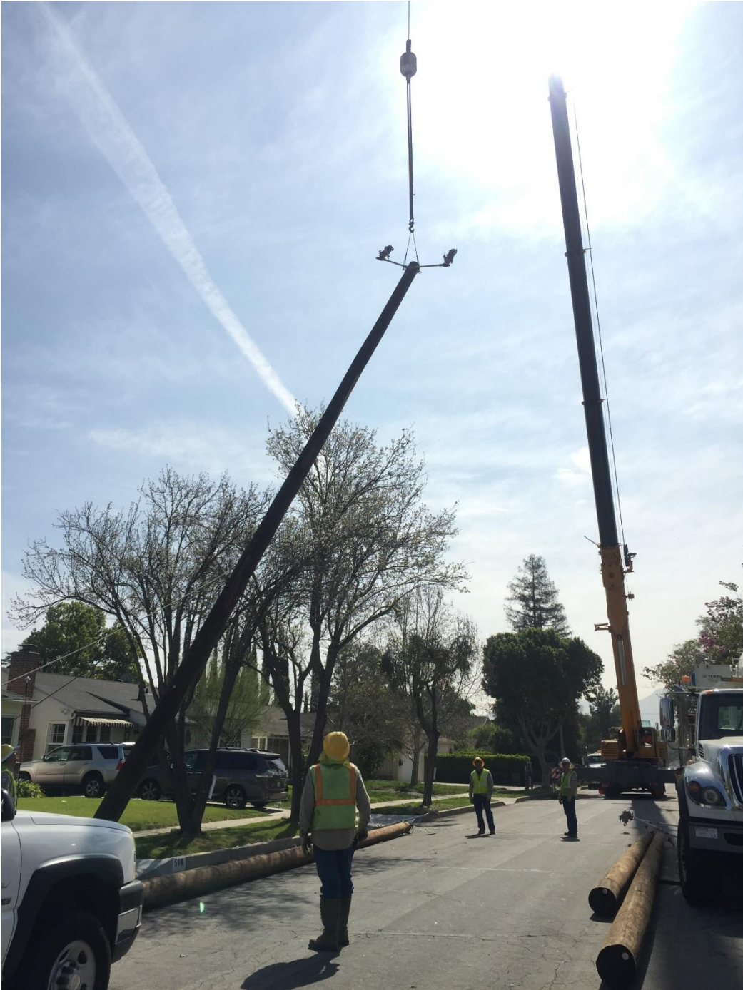
N-15 Property Line – Crane Pole Sets
