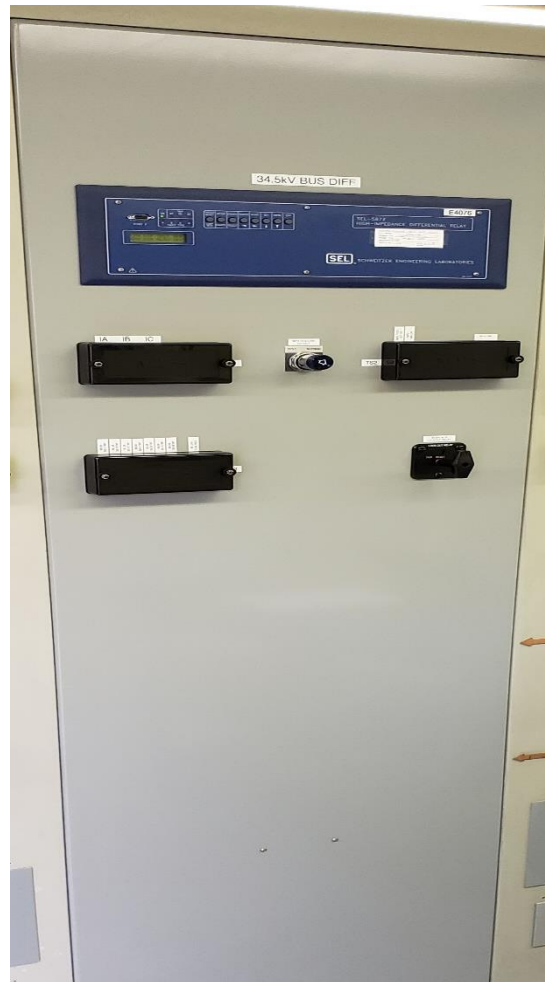
Bus Diff. Relay after Replacement
