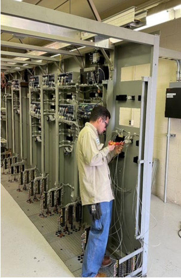
Lincoln-Valley Line new relay during construction at Lincoln
