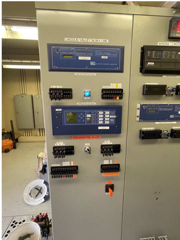
Lincoln-Valley Line new relays at Lincoln
