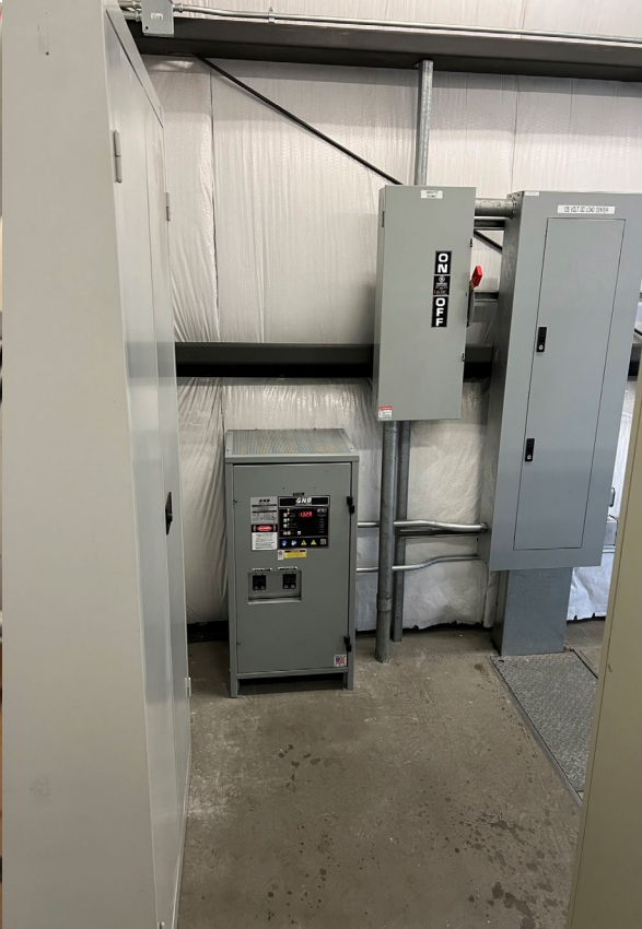
New Charger at Olive GIS Station
