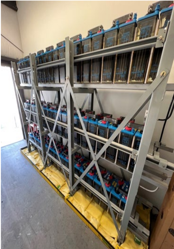
New Batteries at Olive GIS Station
