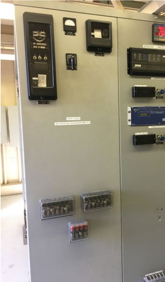
Lincoln-Valley Line old relays at Lincoln
