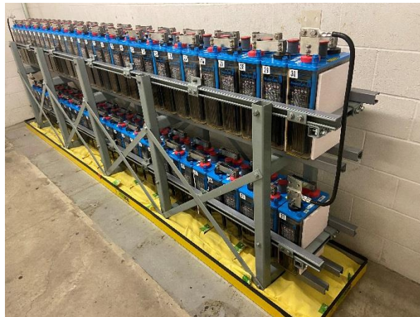
Battery Bank - Installation
