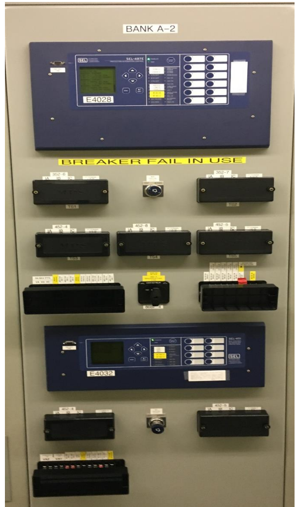
After Installation (New Relays)
