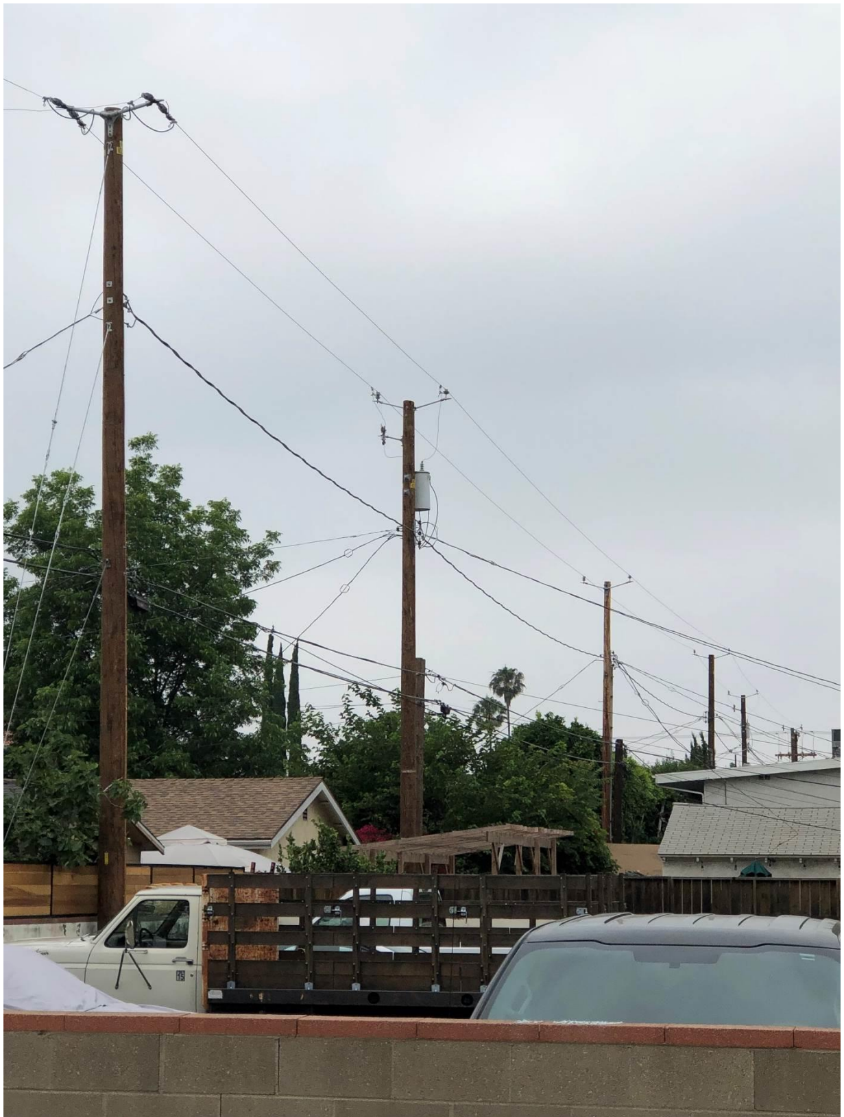
Property Line 12kV Rebuild
