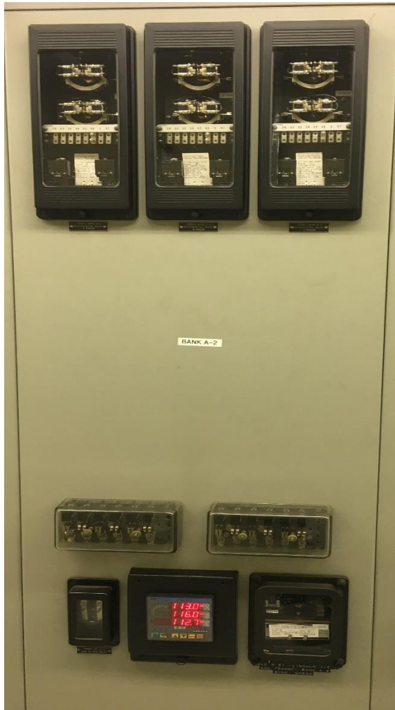
Before Installation (Old Relays)
