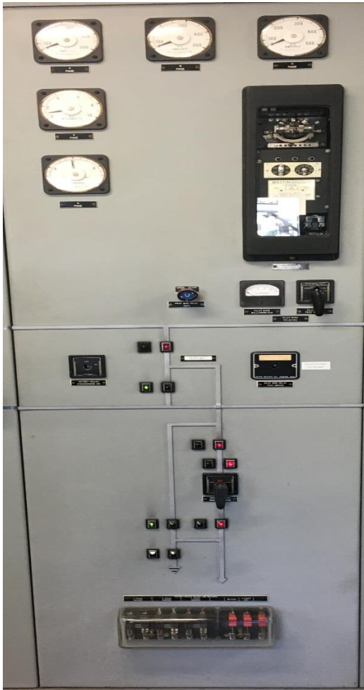
Valley End: Before Installation
