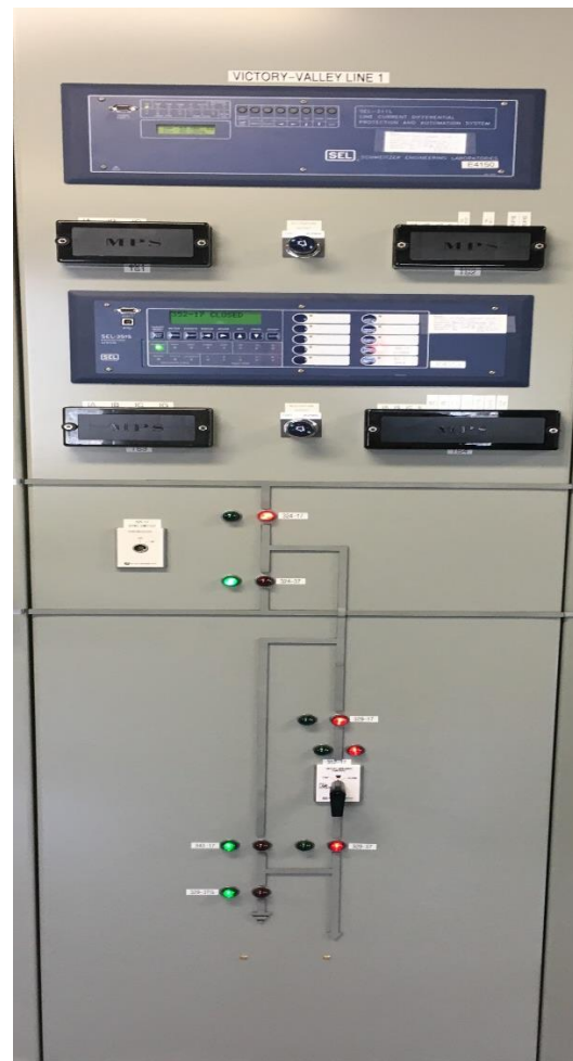
Valley End: After Installation
