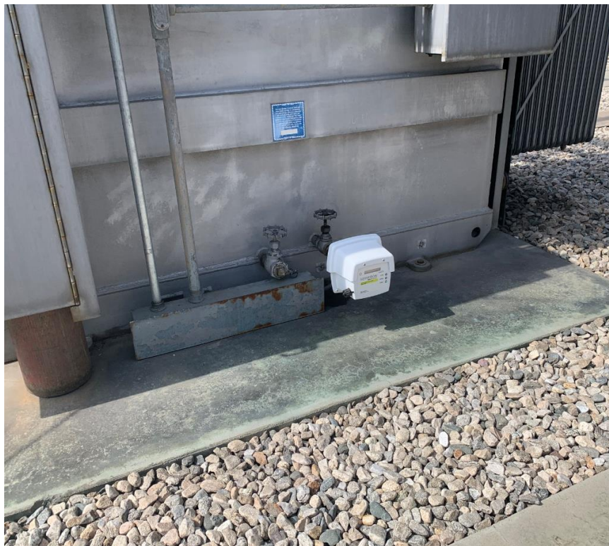
Winona Transformer Bank A-3 Gas Monitor
