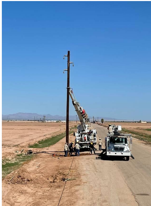
Figure 4 – BWP crew installing a new pole after clear-out of road
