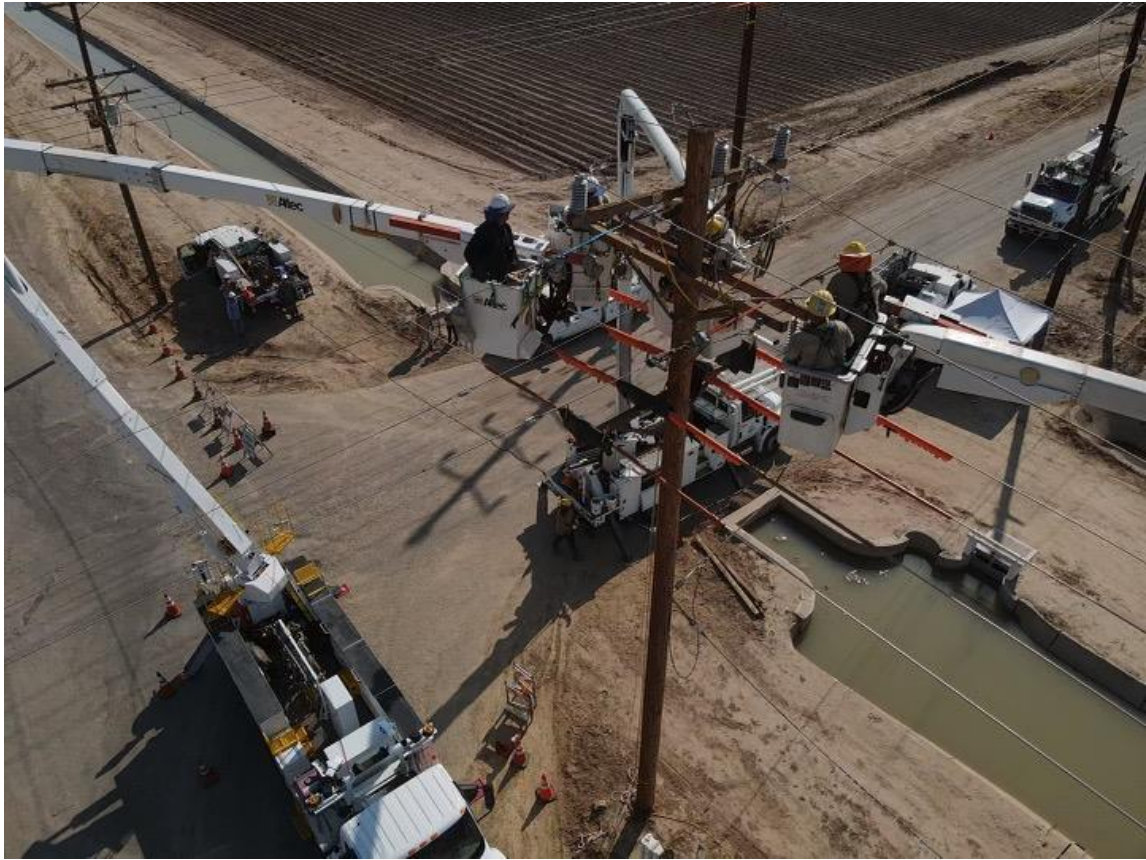
Figure 5 – BWP crew working with other supporting crew on a new pole installation
