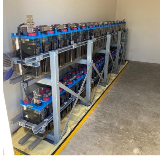
Battery Bank – After Installation
