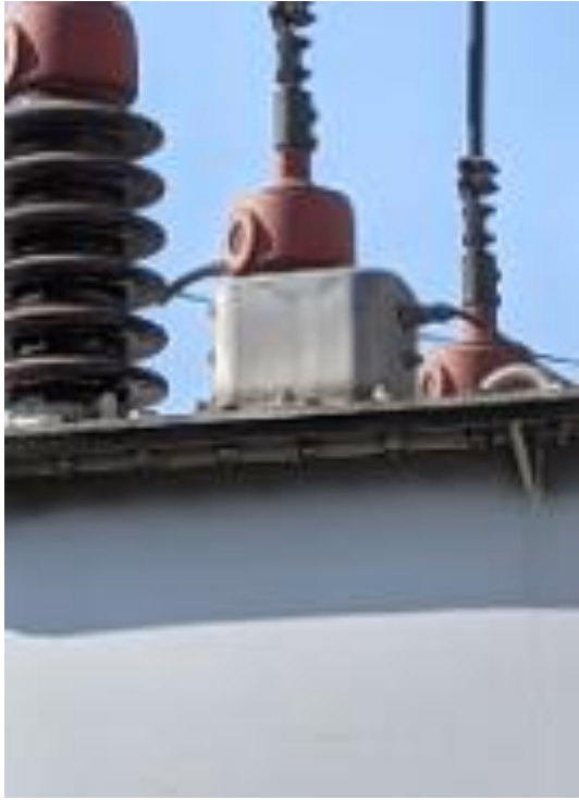
Original Sudden Pressure Relay at Town Bank A-2
