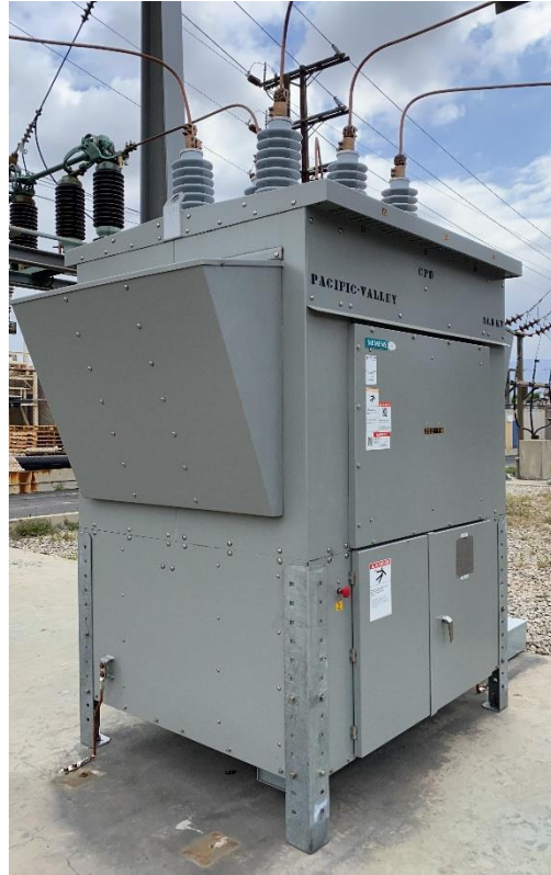
New 34.5 kV Vacuum Circuit Breaker at Valley
