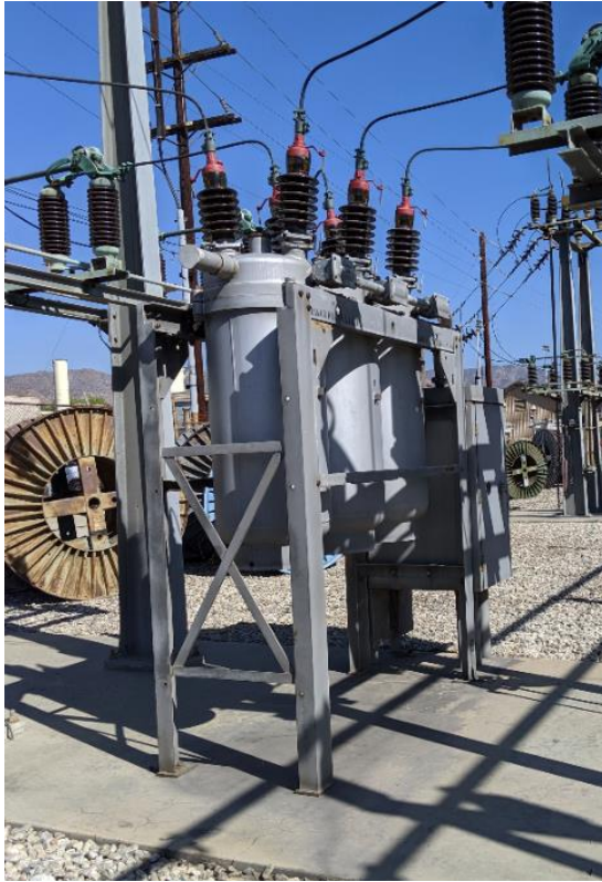
Original 34.5 kV Oil Circuit Breaker at Valley
