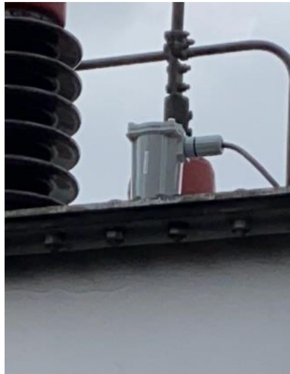
New Sudden Pressure Relay at Town Bank A-2
