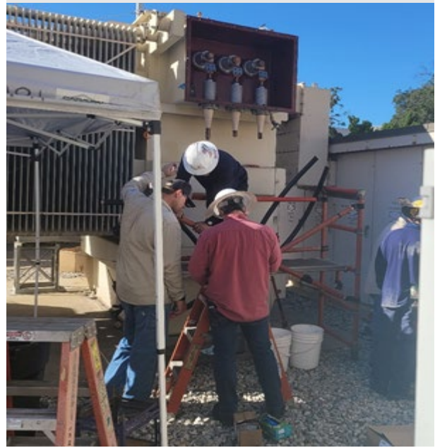
During termination replacement
