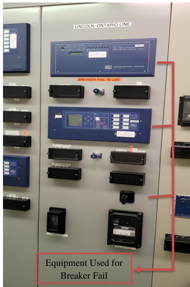
4527 Breaker Fail Addition @ Lincoln Substation
