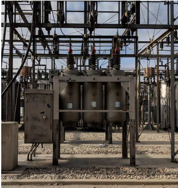
Original 34.5 kV Oil Circuit Breaker
