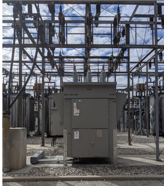
New 34.5 kV Vacuum Circuit Breaker
