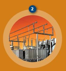
The first stop for the electrical current is a substation where large transformers increase ("step up") the voltage to push the power long distances.
