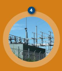
The electricity reaches another substation where the voltage is lowered ("stepped down") so that it can be sent on smaller, distribution power lines.
