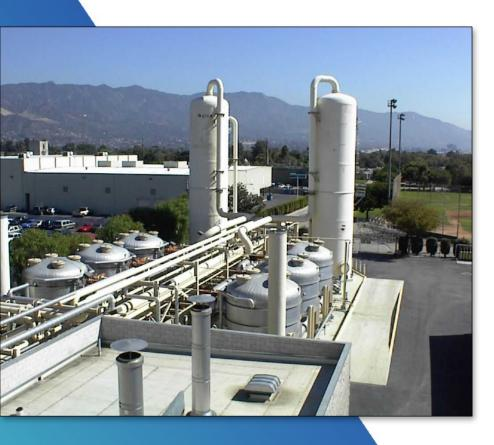
Treats the groundwater to remove chemicals from Lockheed's airplane manufacturing operations
