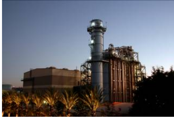
Magnolia Power Project
