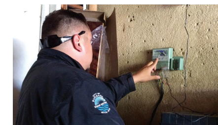
Danny programming a customer's sprinkler system
